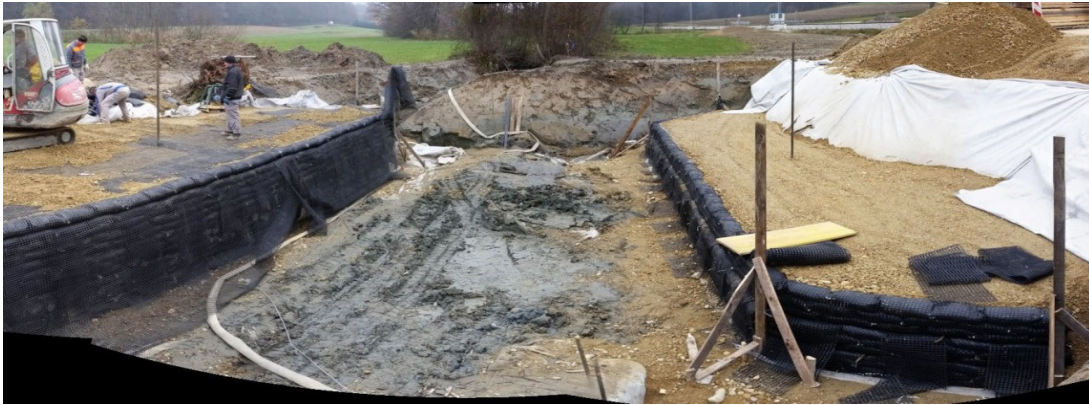
Fig. 5: Construction of the GRS bridge abutments
