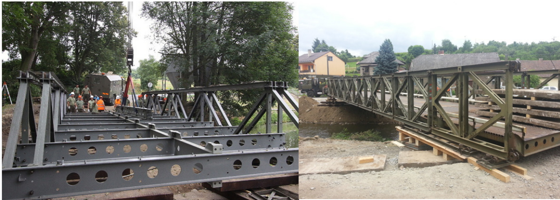
Fig. 2. Assembling of the bridges.
