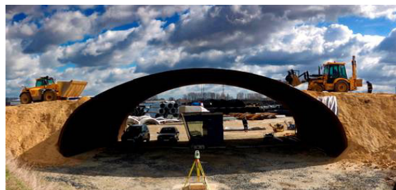
Fig. 1. The SuperCor SC-57S structure in the construction phase
