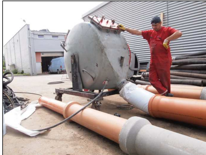
Fig. 1. Inversion drum during liner installation.
