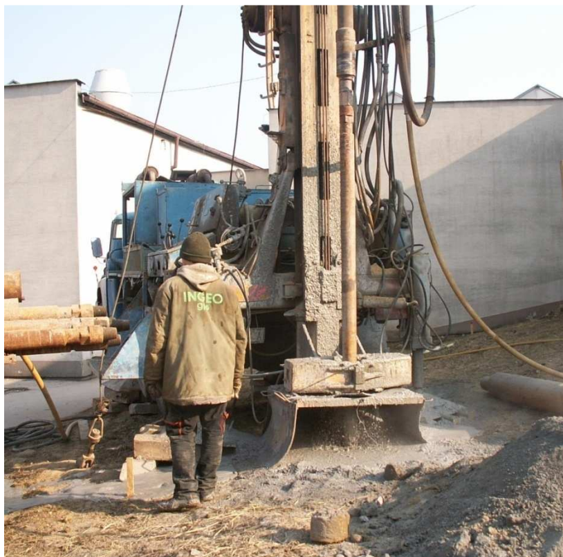
Fig. 3. Sinking geothermal borehole.
