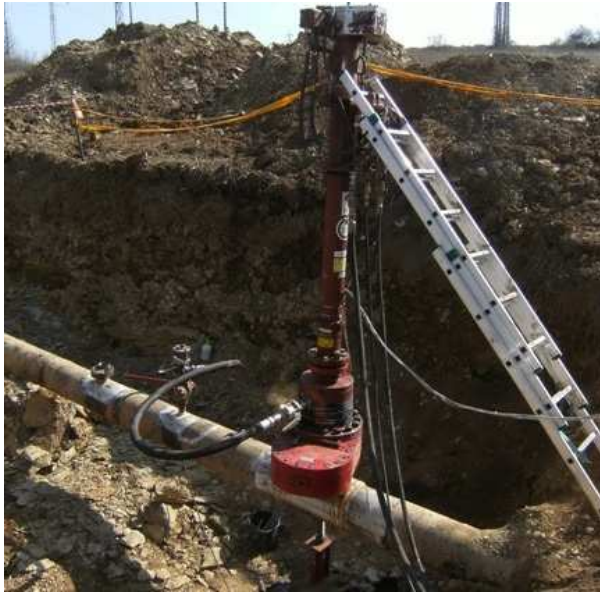
Fig. 6. Course of drilling a hole in gas pipe and behavior of beginning measurement of torque.
