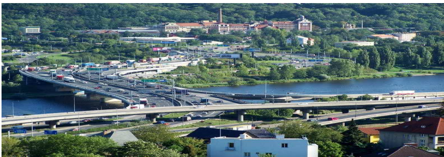
Fig.2 Road transport infrastructure
